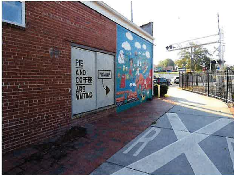
Exterior of Building as of September 2022
