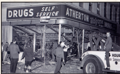
Atherton Drug Store natural gas explosion: October 31, 1963
