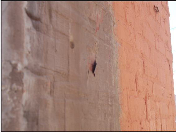
Figure 7.2: This masonry has been inappropriately painted, causing the paint to peel off within one year of its application. The painting of masonry can cause recurring maintenance issues and may cause damage to the masonry.
