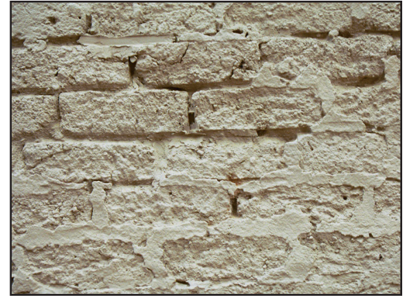
Figure 7.1: This is an example of what happens when masonry is cleaned improperly by sandblasting of the surface. Masonry has a protective "skin" which protects against infiltration of moisture. If this skin is removed, as is the case with sandblasting, the brick can no longer repel moisture.
