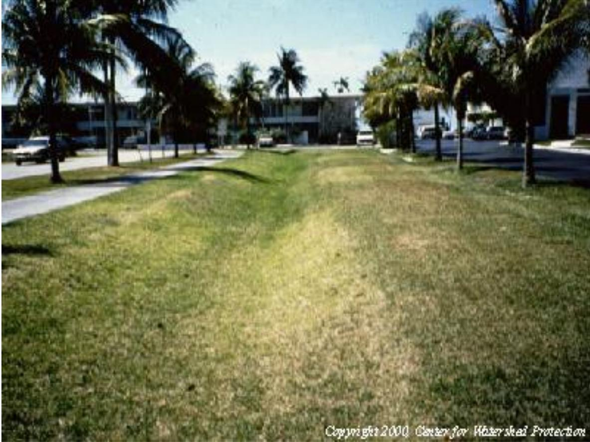
*Above: dry swale for filtration;      Below: Wet swale for water quality*
